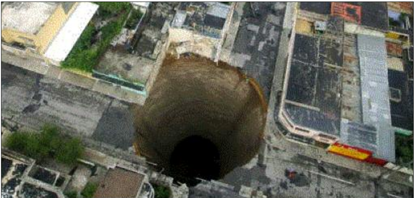
The Guatemala City sinkhole of 1 June 2010 (Source: Casa Presidencial handout)
